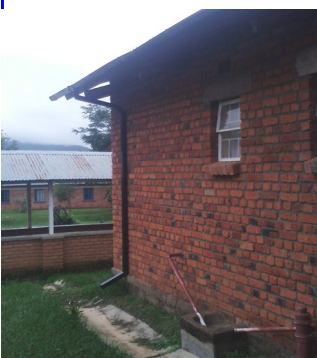
Gutters at premises
